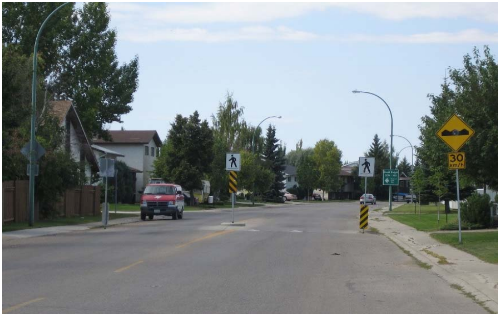
Exhibit 5-8: Mellicke Road between David Knight Crescent and Stechishin Crescent (Silverwood Heights)
