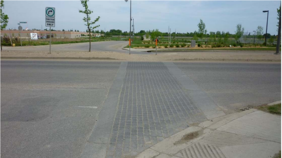
Exhibit 5-10: Textured Crosswalk using pavers at Stonebridge Boulevard and Wellman Crescent (Stonebridge)
