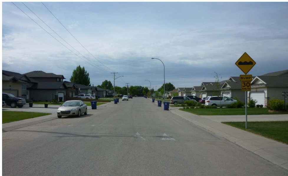
Exhibit 5-11: Speed Hump on Hughes Avenue (Dundonald)
