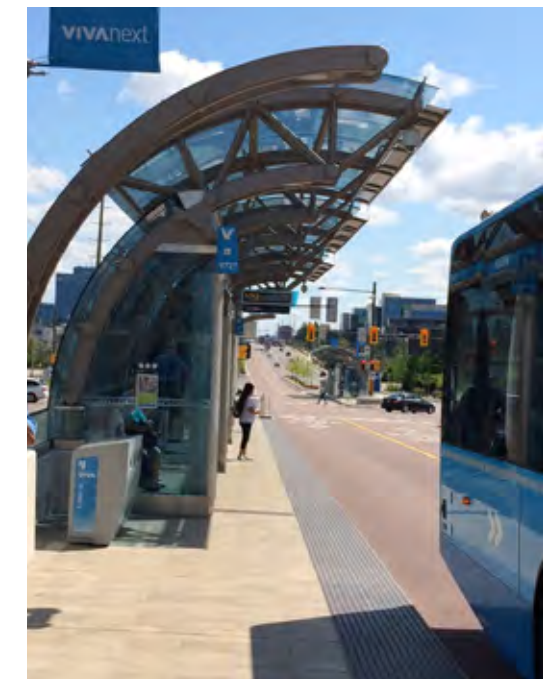
Figure 4.02 - Completed BRT Station
