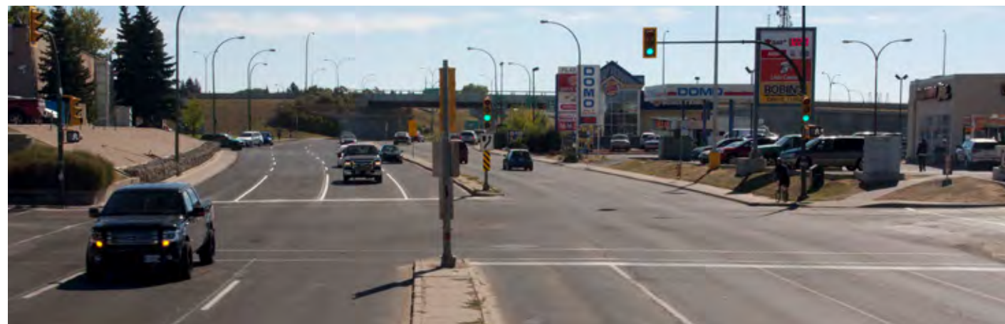
Figure 2.52 - Confederation Drive at Confederation Suburban Centre (looking south)
