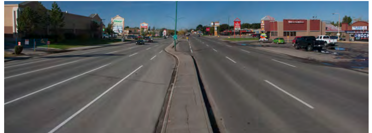
Figure 2.26 - 8 th Street Existing Condition
