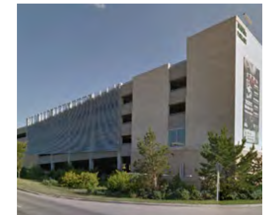
Figure 2.40 - Existing Parkade adjacent to College Drive
