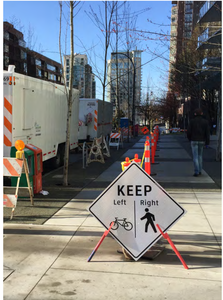
Construction Detour, Vancouver, BC, Source: Urban Systems
