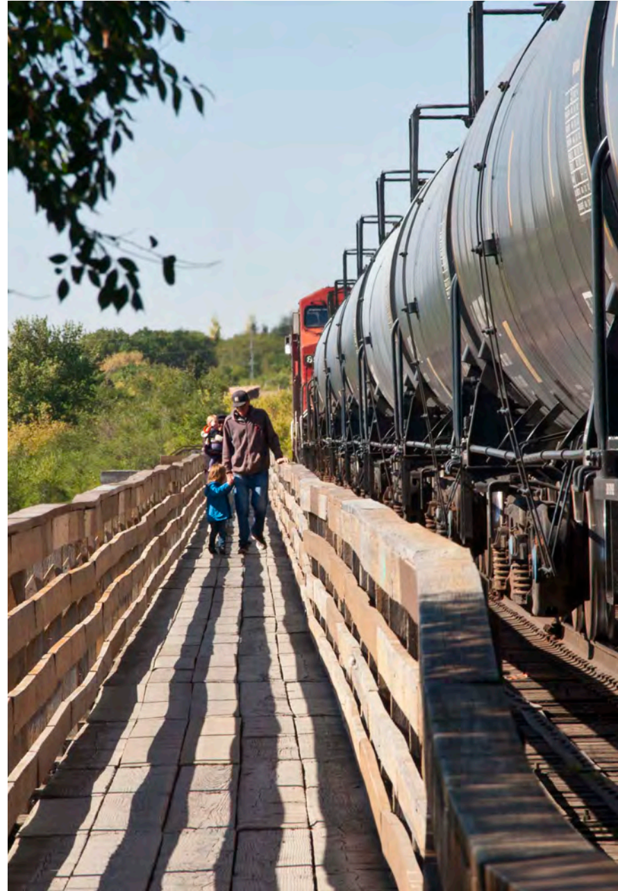
CRP Rail Bridge, Saskatoon, SK, Source: Urban Systems
