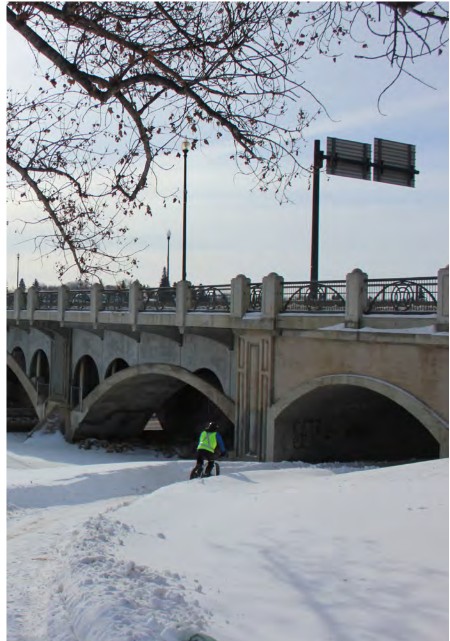
Broadway Bridge Underpass, Saskatoon, SK, Source: Urban Systems
