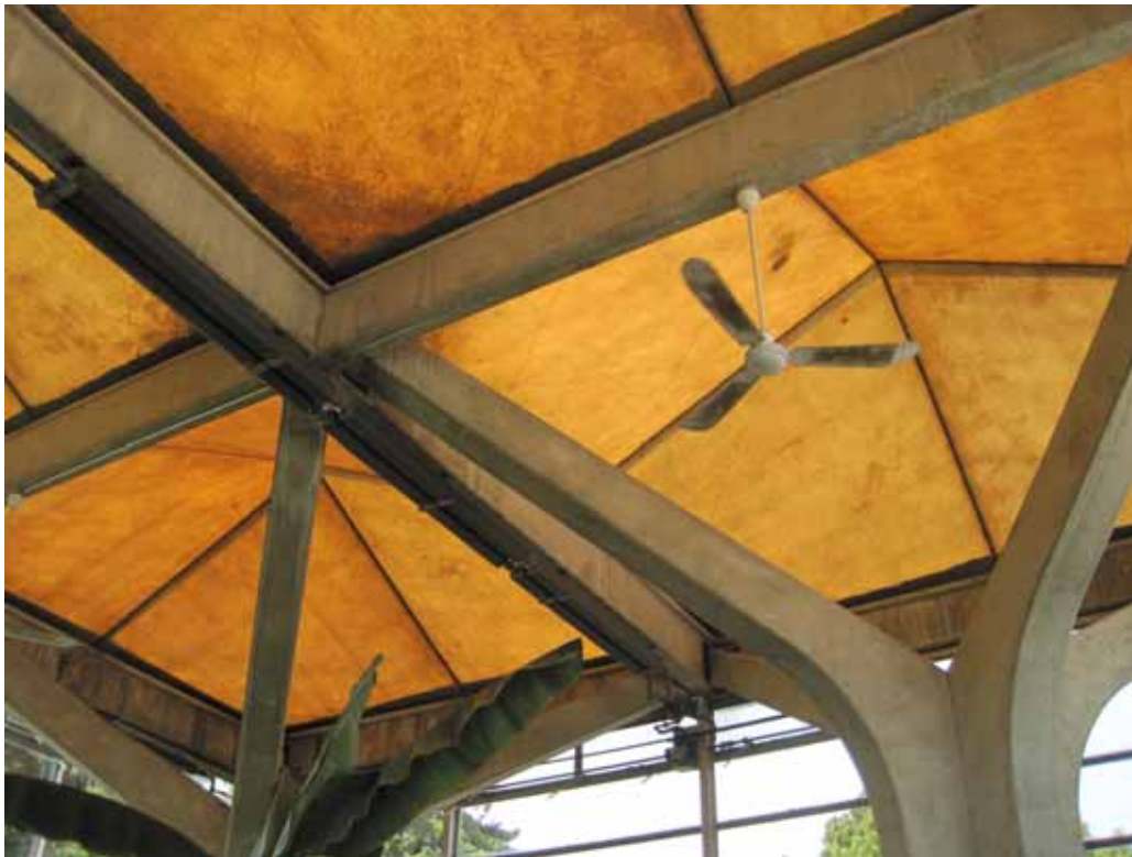
PHOTOGRAPH NO. S11-7721A-06 Conservatory (roof).
