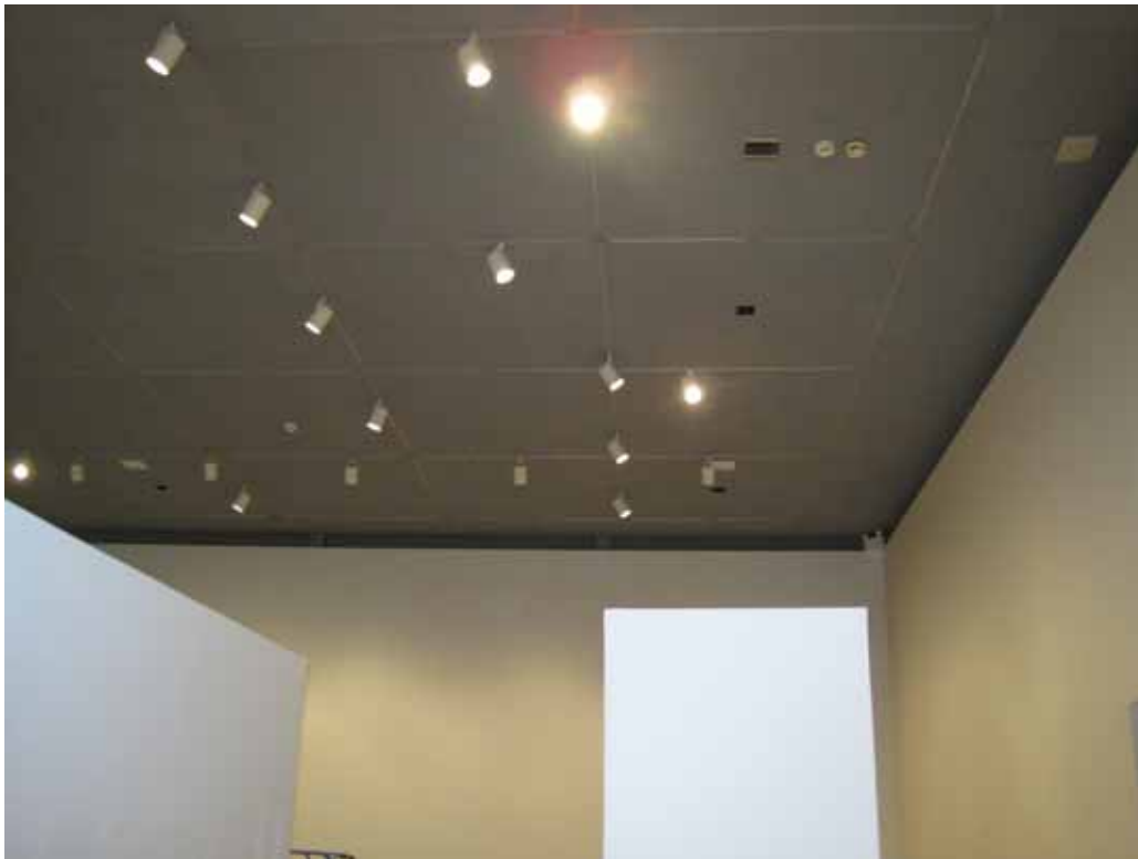
PHOTOGRAPH NO. S11-7721A-07 Art gallery area.
