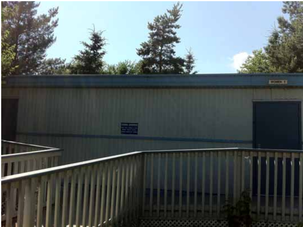
PHOTOGRAPH NO. S11-7721A-15 Washrooms.
