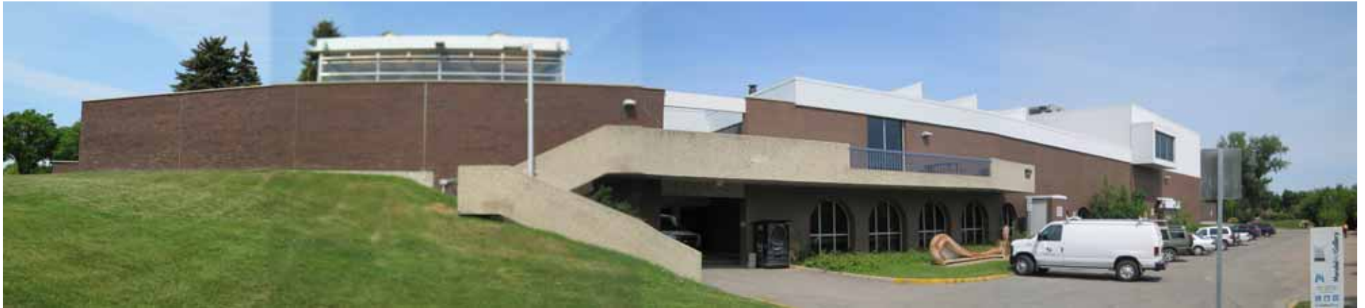
PHOTOGRAPH NO. S11-7721A-03 Panoramic photograph taken proximate the southeast side of the subject property looking west to north.
