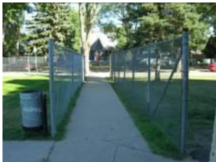
Possible entrapment area where a 2nd layer of fencing has been placed along sidewalk.
