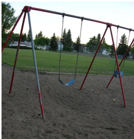
Play equipment in need of paint
