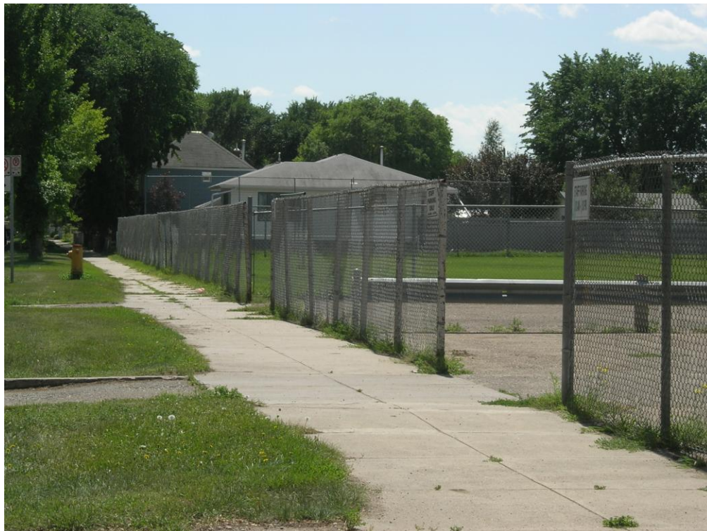
Openings in the fencing are difficult to see
