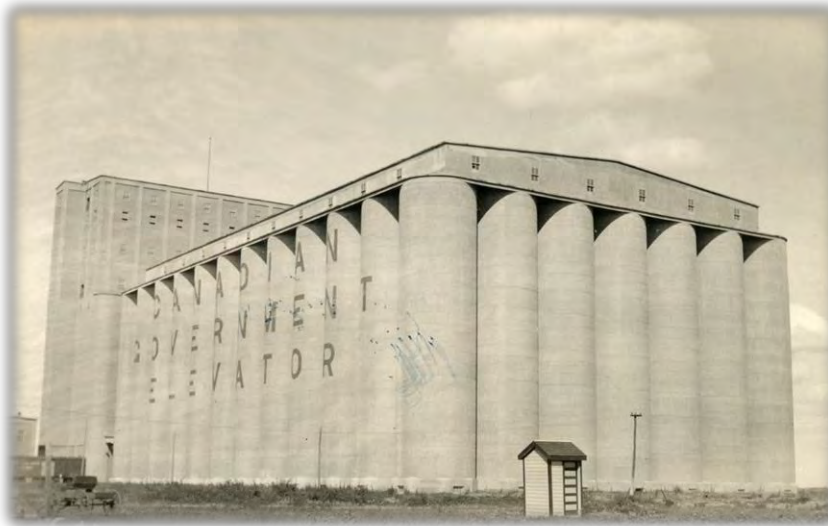
Canadian Government Grain Elevator – 1920 (credit: Photograph LH-7381-A by Unknown, courtesy Saskatoon Public Library – Local History Room)
