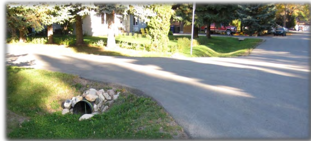
Ditch & Culvert (Majority of Montgomery Place)
