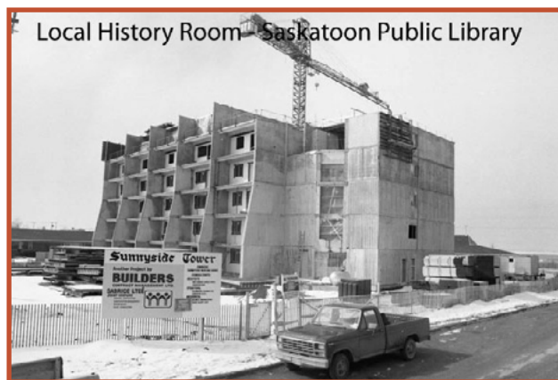
Sunnyside Tower under construction on Hilliard Street West and St. Henry Avenue.
