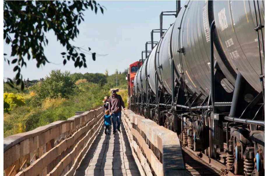
CRP Rail Bridge, Saskatoon, SK, Source: Urban Systems
