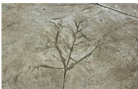
Plants imprinted on concrete
