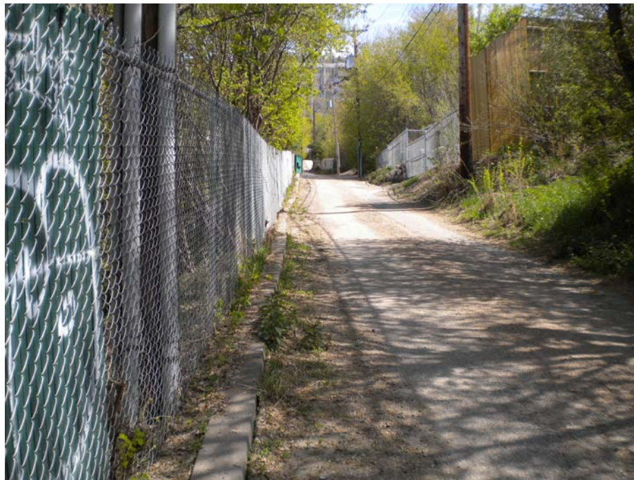
Photo C.2. Looking East at Deflection of Curb and Fence Line along Cherry Lane (May 27, 2010)
