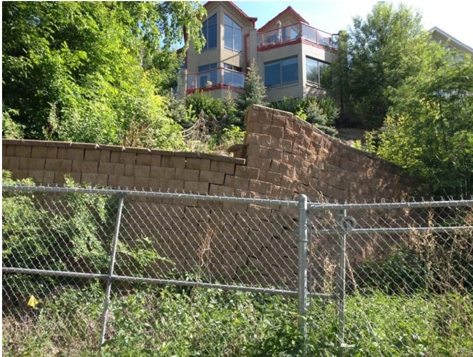
Photo C.17. Retaining Wall in Backyard of 237-239 11th St. E. (June 4, 2013)
