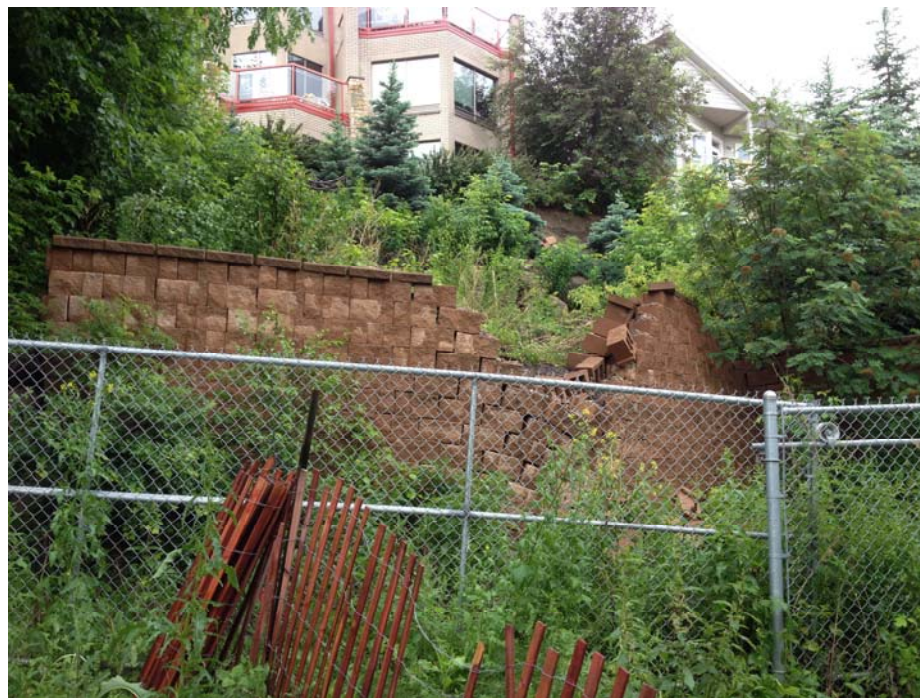
Photo C.18. Retaining Wall in Backyard of 237-239 11th St. E. (June 20, 2013)
