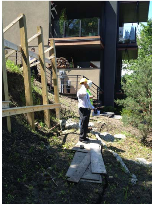
Photo C.11. Cracking along Headscarp of East Failure (June 21, 2012)
