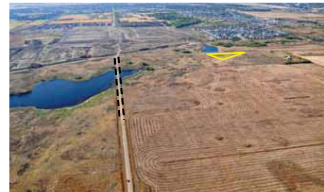
Crossing #3 Detail (Looking South)
