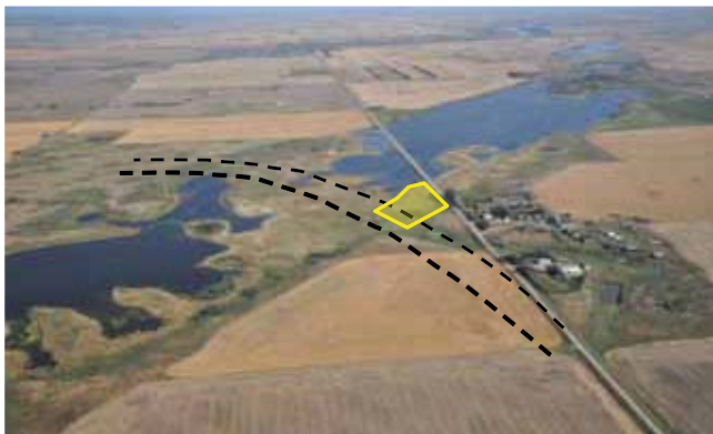
Crossing #1 Detail (Looking North)
