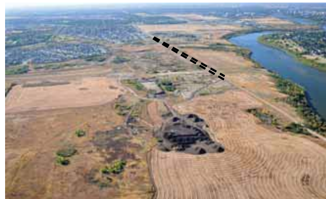
Crossing #2 Detail (Looking South)
