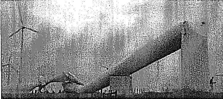
Turbine Structural failure in Western Germany
