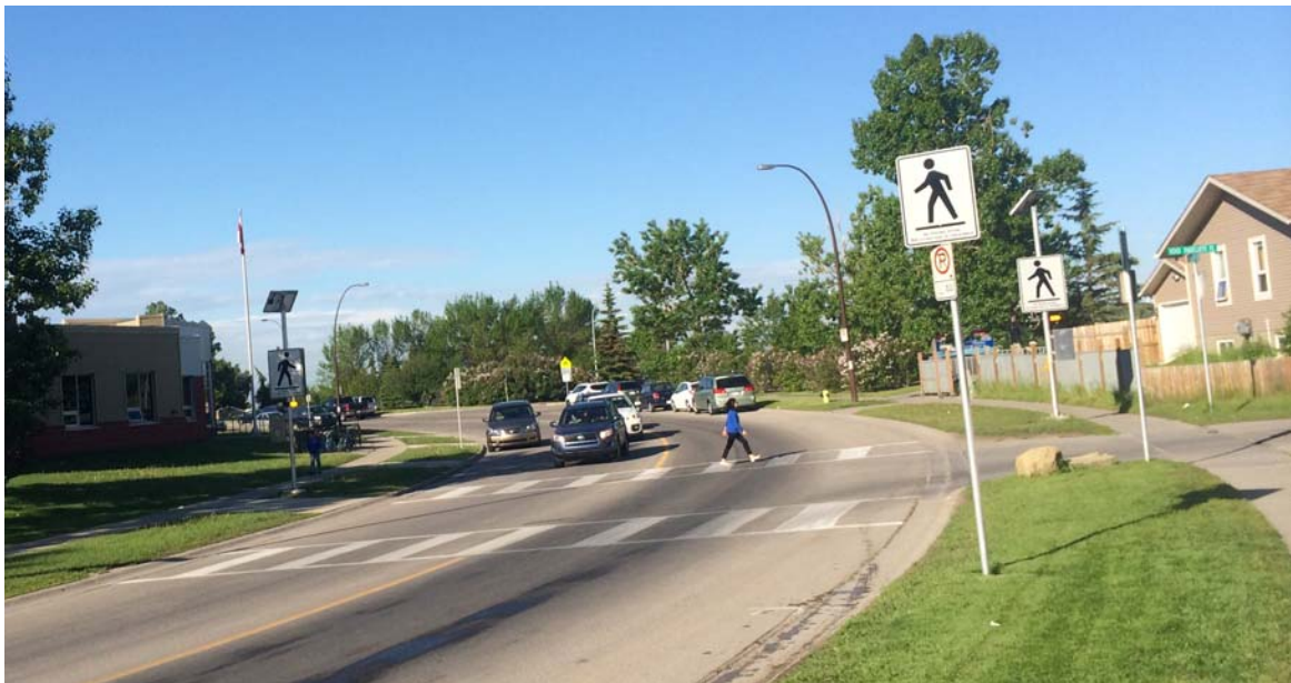
Figure 3: RRFB installed in a School Zone 15
