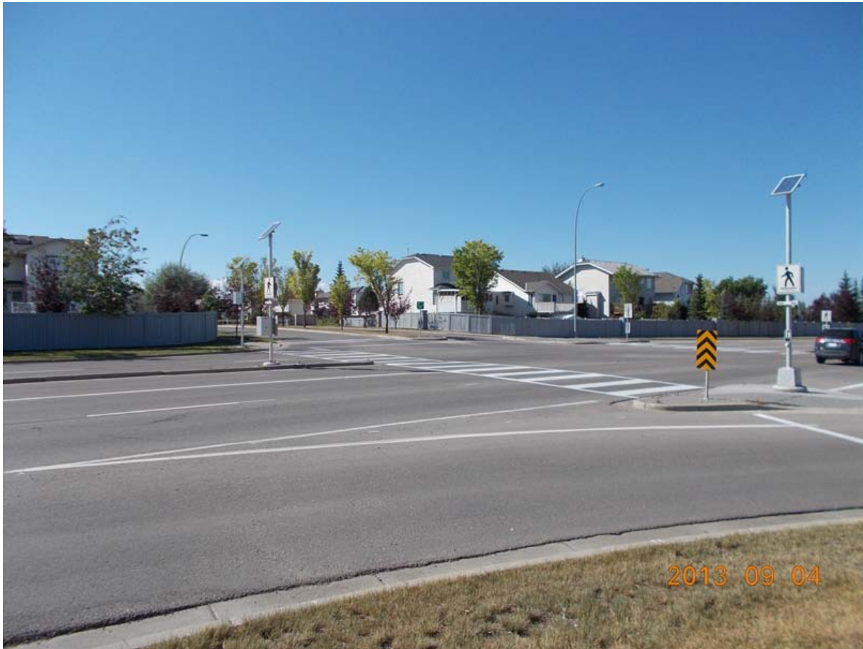
Figure 2: Typical RRFB Installation 1
