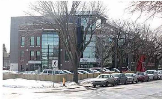
Wilson School is now home to Affinity Credit Union (Photo by Sandy Hutchinson)
