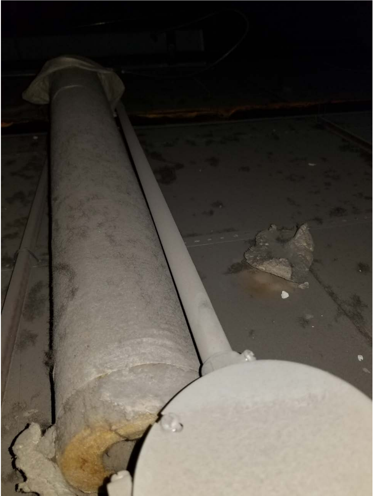
Figure 2. Fibreglass Pipe Insulation Laying on Ceiling Surface.
