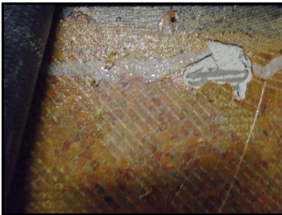
Photograph 3: Asbestos-Containing Vinyl Sheet Flooring, Orange and Red.
