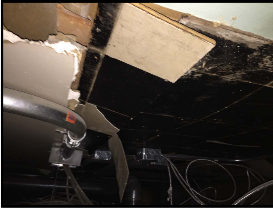
Photograph 3: Asbestos-containing 9"x9" Floor Tile on Upper Plywood Ceiling.
