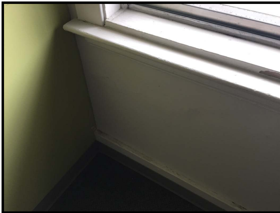
Photograph 5: Asbestos-Containing Plaster.
