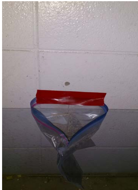
PHOTO 2 – 124 (BAY #10) - EAST BLOCK WALL
