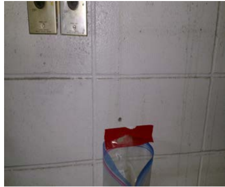
PHOTO 1 – 124 (BAY #10) – NORTH BLOCK WALL
