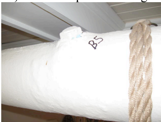
#5) Mud Compound Fitting
