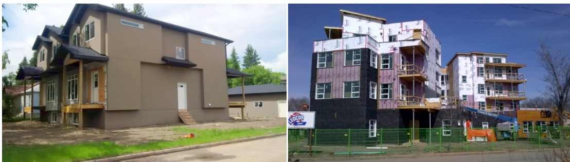
Typical semi-detached infill project in an established neighbourhood (left), and a new multi-family condominium project in an established mixed use neighbourhood (right).
