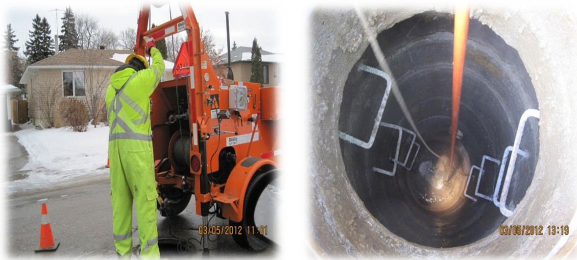
Figure 36: Photographs of Closed-Circuit Television Inspection Work
