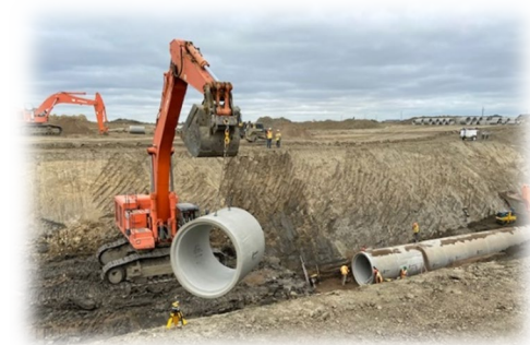
Figure 42: Brighton Storm Trunk Installation
