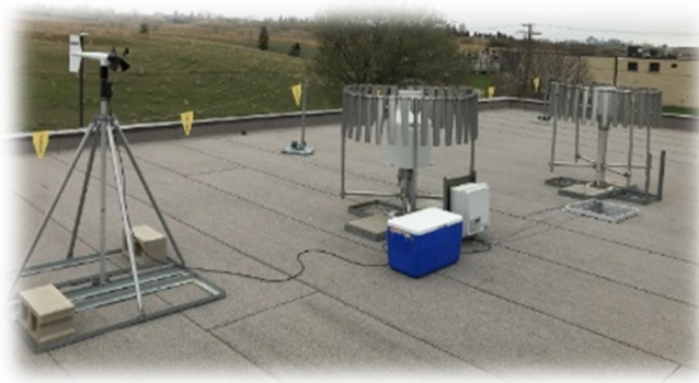
Figure 40: Photograph of Rainfall and Wind Measurement Equipment
