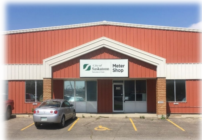
Figure 3: Photograph of the Meter Shop
