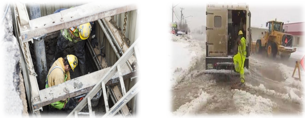
Figure 33: Photographs of Water Main Break Repair Work
