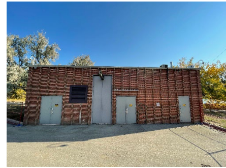
Figure 37: Spadina Lift Station
