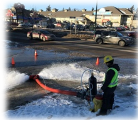
Figure 41: Fire Flow Testing
