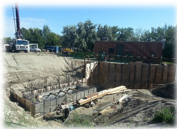
Figure 5: Photograph of Lift Station Infrastructure Construction
