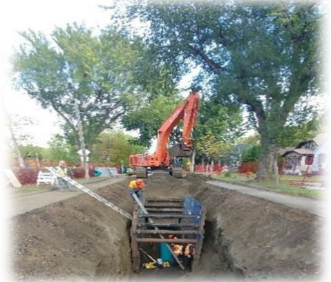
Figure 7: Photograph of Work in an Excavated Trench
