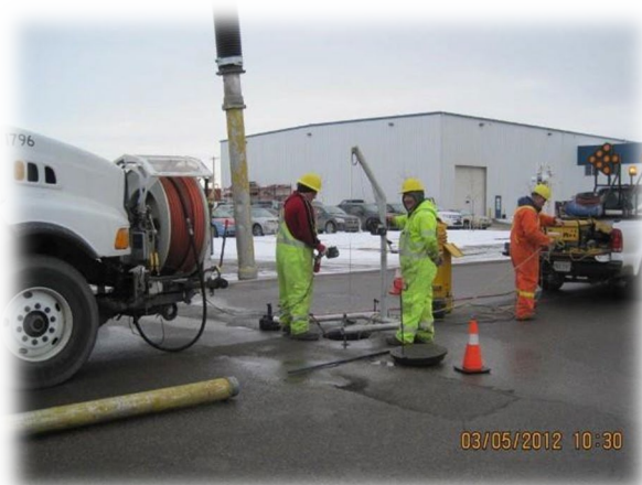
Figure 6: Photograph of Sewer Inspection Activities
