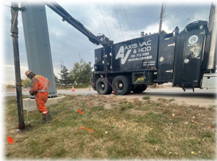
Figure 6: Hydrovac Work for the CN Industrial Drainage Improvement Project
