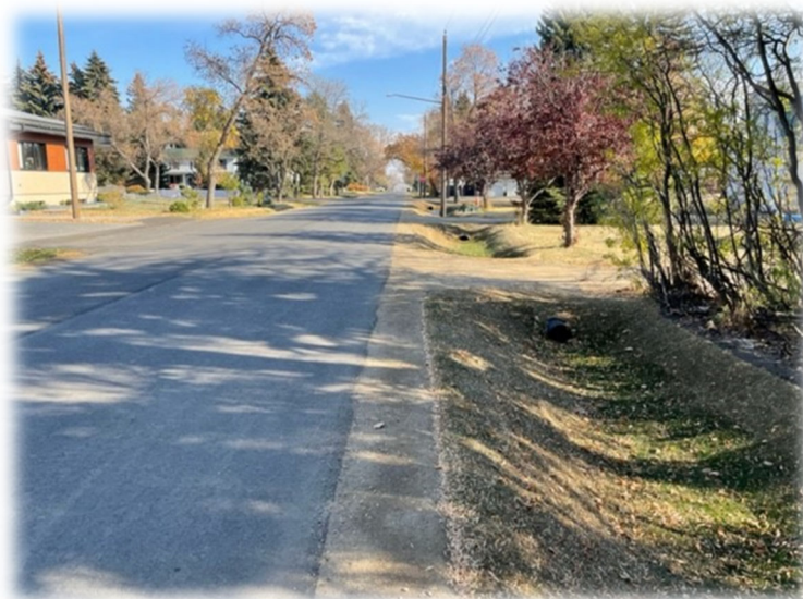
Figure 5: Completed Ditch Improvements in Montgomery Place
