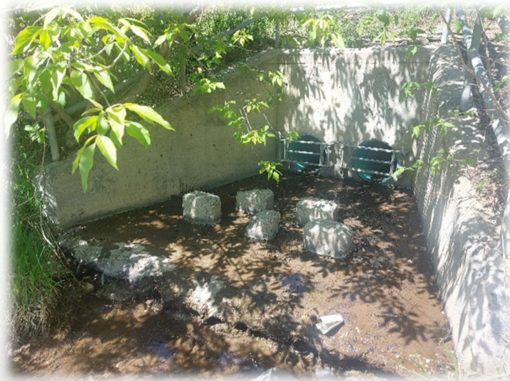
Figure 1: Storm Water Outfall Structure Along the South Saskatchewan River
