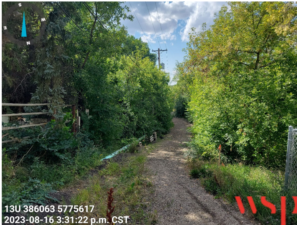
Photograph 1: Looking west down the back alley at the East Failure (August 16, 2023)
