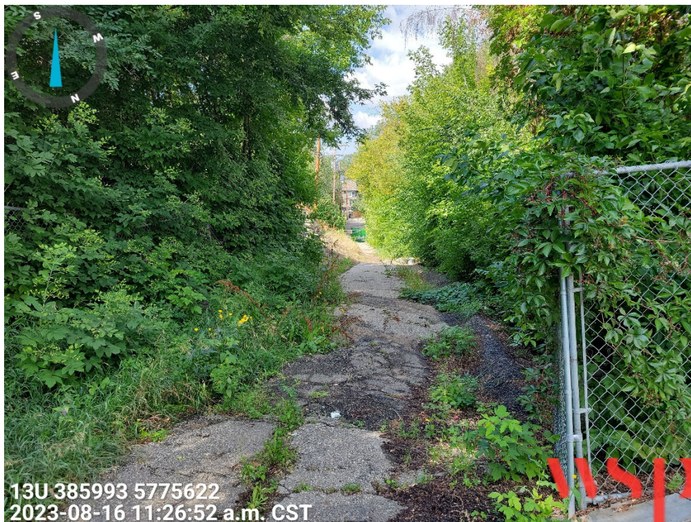
Photograph 2: Looking west down the back alley at the West Failure (August 16, 2023)
